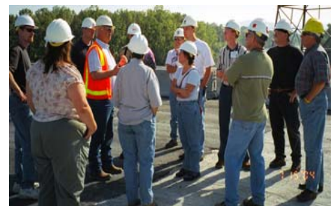
Jim Sly (4th from left) of Hamilton Construction Co. explains bridge-building to Eugene teachers on the I-5 bridge
