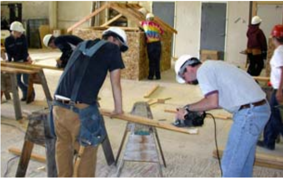
Cutting rafters for mini-structures at the Willamette Carpenters Training Center
