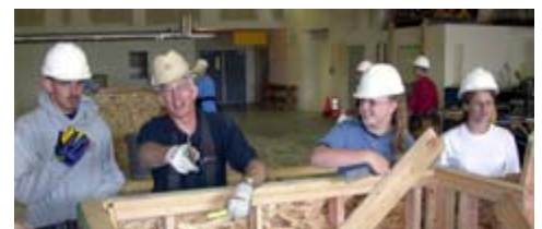
Jim Murphy shows Construction Academy students how to build a mini-structure at the Willamette Carpenters Training Center.
