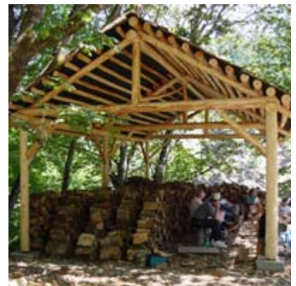
Pole barn on the Rogue River built by Construction Academy students led by teacher Doug Gardner of Crater High School.
