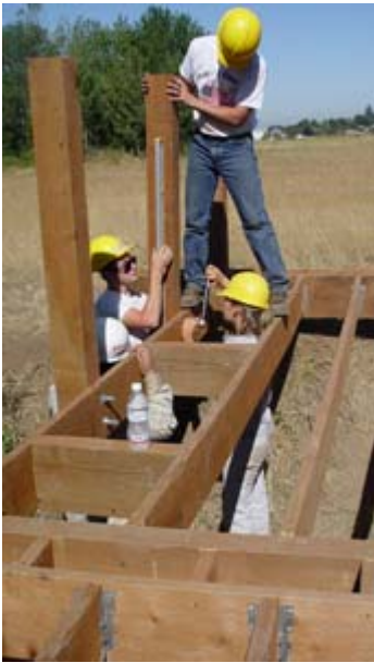
Bridge construction at the Molalla wetlands.
