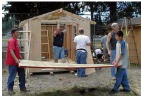
...and carpenters raise high the roof beam...
