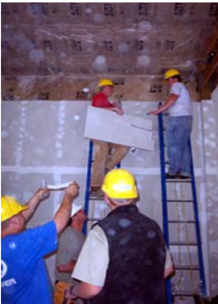
Clackamas sheetrock team in action.
