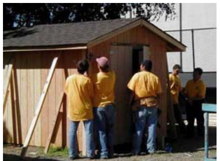
... until the building is complete.
